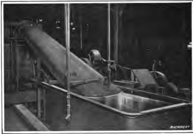
Fig. 15. Delivery End of Gas Medium Furnace—Note Arrangement of Water Seal
